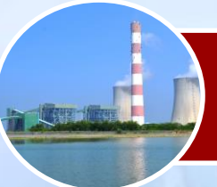
Jaypee Nigrie Super Thermal Power Plant 2X660 MW
