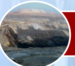
Amelia (North) Coal Mines 3.36 MMTPA Mining Capacity
