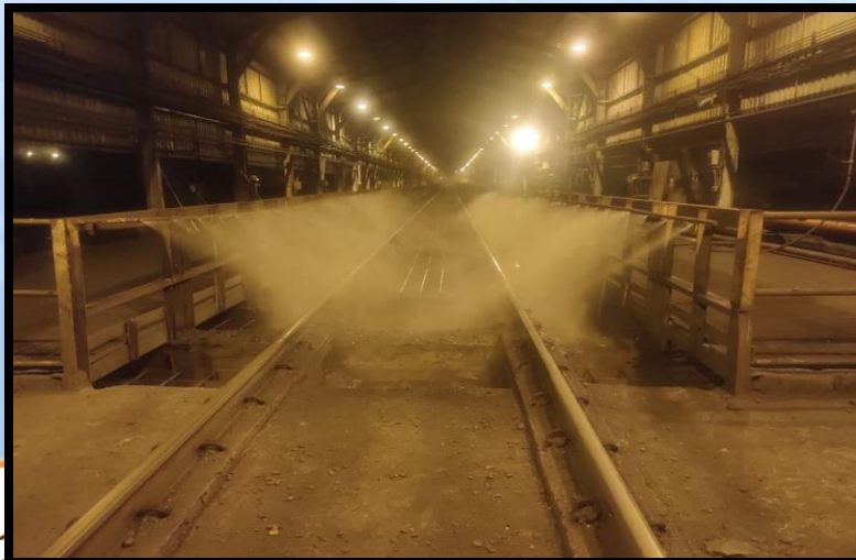
Water fogging system at Track hopper
